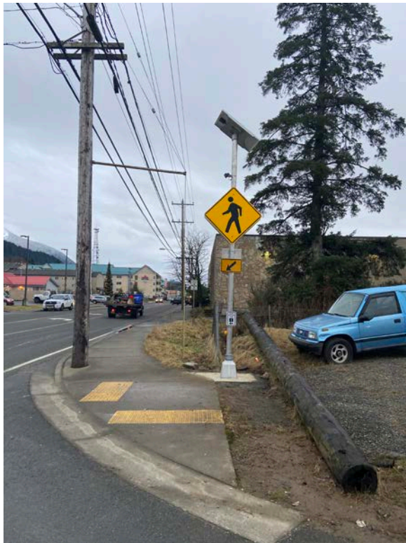
New Push Button Actuated Pedestrian Signs at Heckman St.
