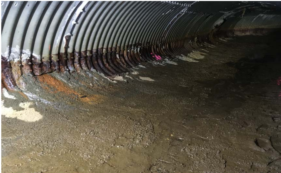
Schoenbar Culvert after Temporary Concrete Placement
